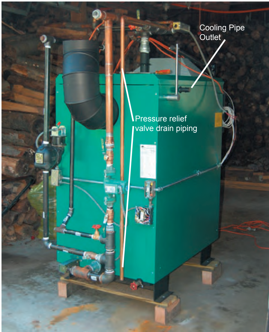
Photograph showing one of the cooling pipe outlets and the pressure relief valve piped to within 6 inches of the floor with rigid copper pipe.
