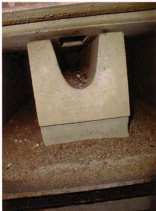
Fig. 4: - view of the boiler combustion chamber
