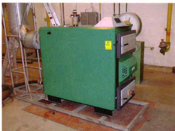
Fig. 2 - overall view of the boiler
