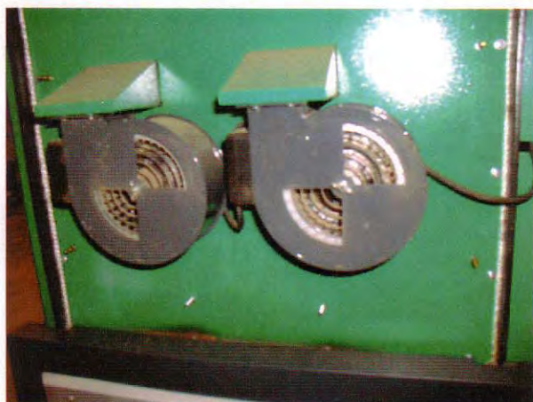
Fig. 3: - combustion air fans
